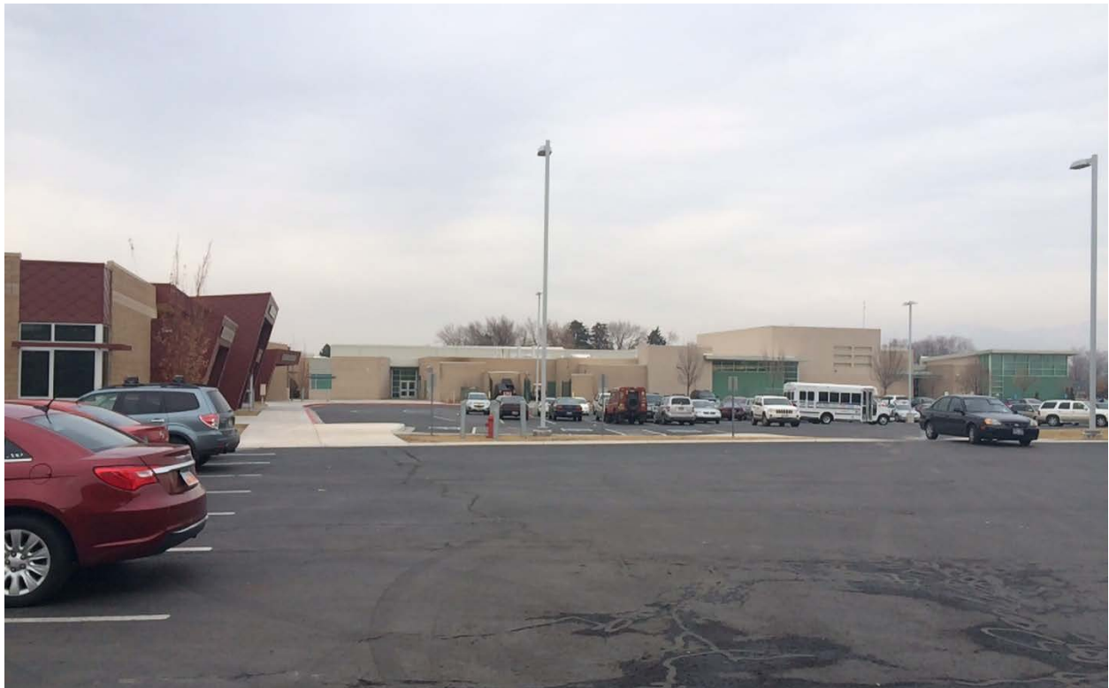
Adjacent land uses to the north of the subject building. Mountain View Elementary School is located north of the building on the same parcel.
