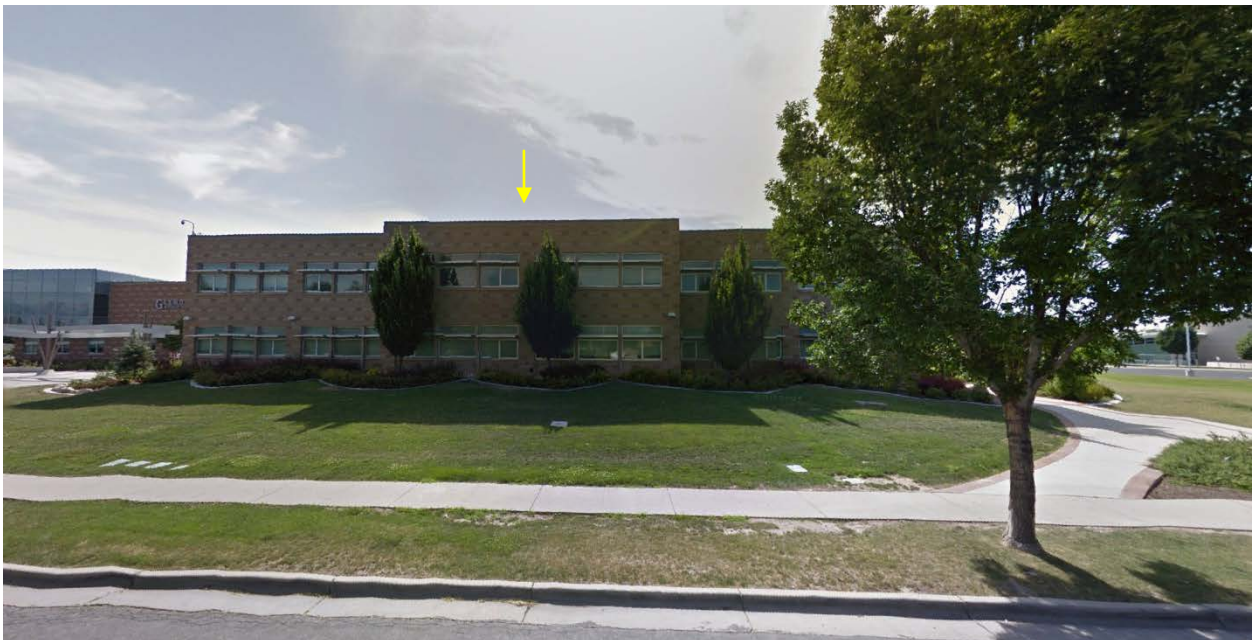
Street view of the east elevation of the subject property from Navajo Street. The proposed location of the antennae adjacent to the east elevation is identified with a yellow arrow. The 8' tall antennae will be set back 19' feet from the parapet wall, minimizing or eliminating visual impact as seen from the public views.
