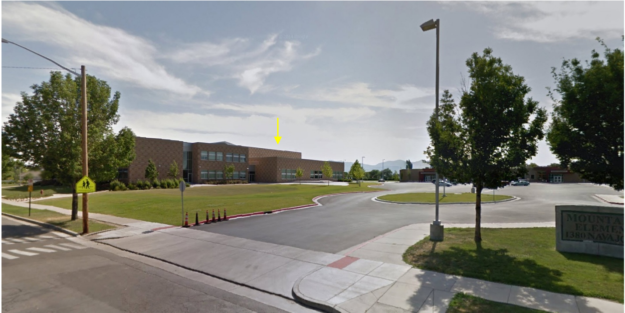
Street view of the north elevation of the subject property from Navajo Street. The proposed location of the antennae adjacent to the north elevation is identified with a yellow arrow. Its proposed location is on the second story and will be set back 15 feet from the parapet wall, minimizing or eliminating visual impact as seen from the public views.
