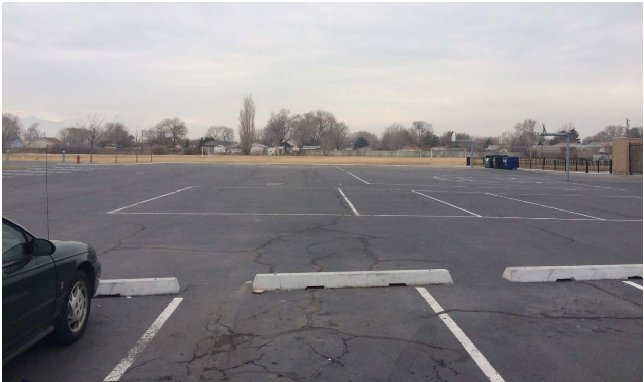
View of adjacent land uses to the west of the subject building. The electrical equipment is proposed on the west side of the building. The parking lot and the recreation fields act as a buffer between the residential uses to the west of the subject property.
