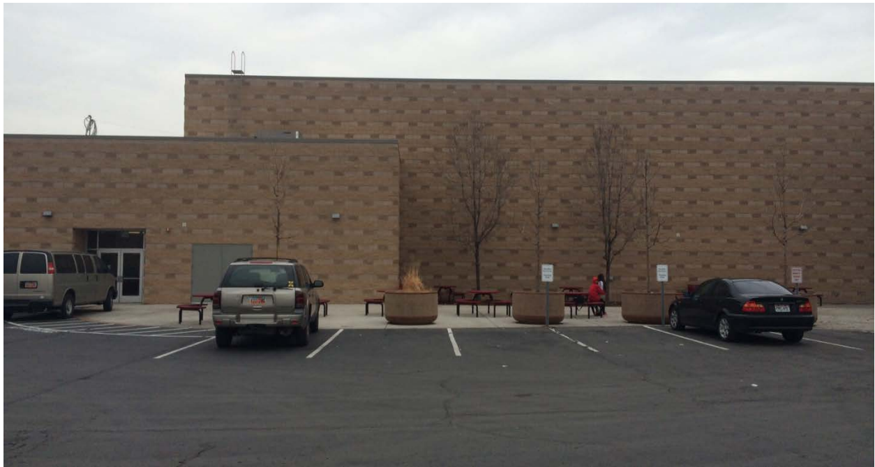
View of the west elevation of the subject where the antennae related electrical equipment is propose adjacent to the building behind a concrete masonry wall that will be constructed out of materials to match the existing building.
